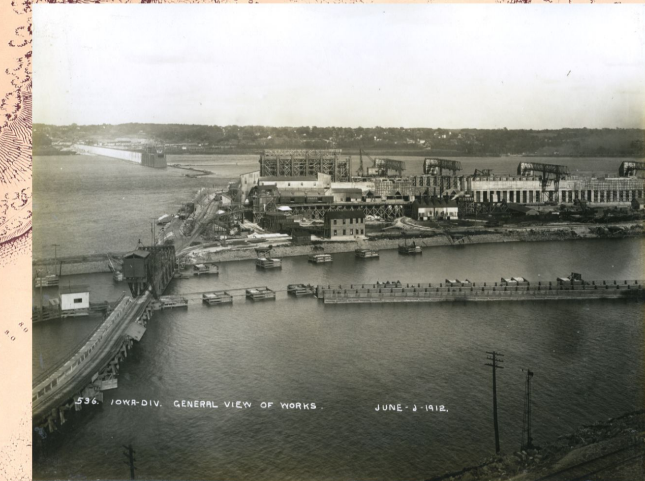
Keokuk-Hamilton Dam under construction Courtesy of Keokuk Public Library, Keokuk, Iowa
